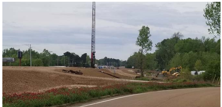
View of the West County Line Road worksite
